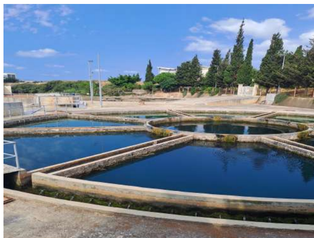
Figure 8: Tripoli Water Treatment Plant
