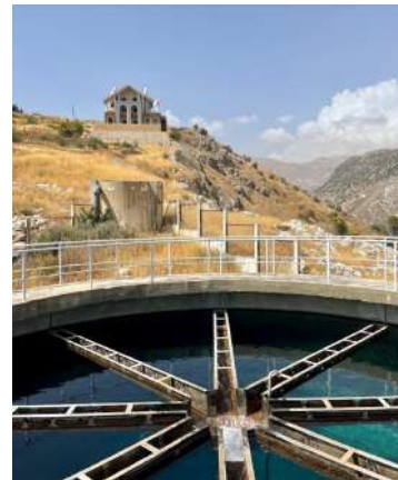
Figure 10: Zahle Water Treatment Plant
